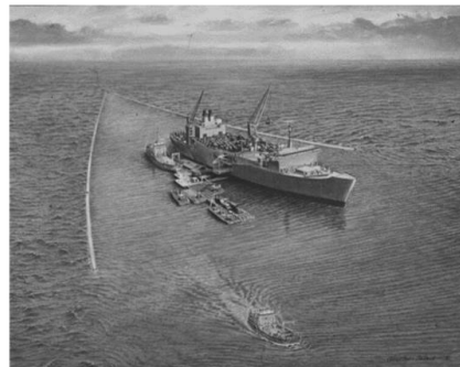
Figure 1. Rapidly Installed Breakwater System (RIBS) concept.
